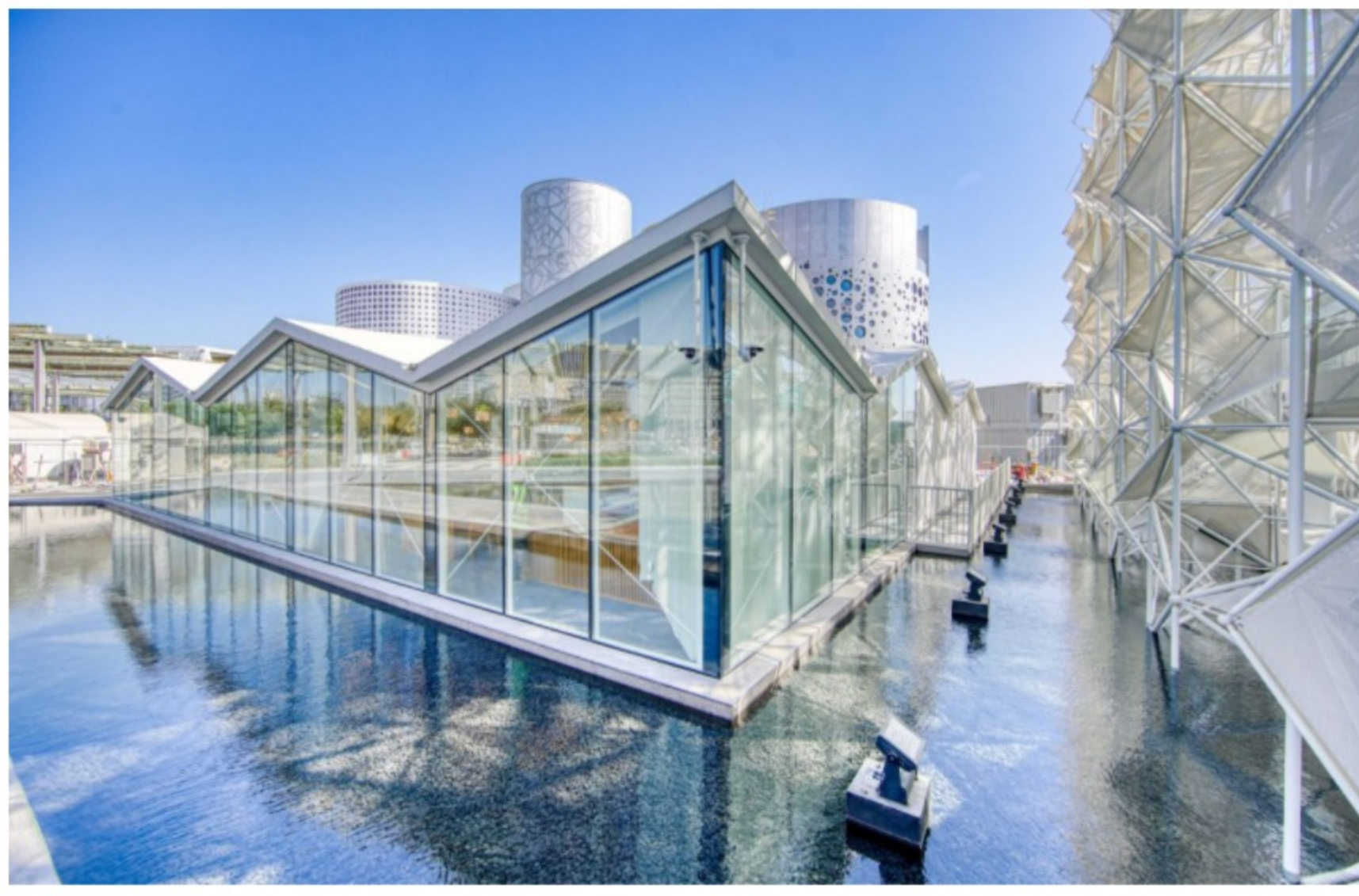
Red Sea Int'l delivers modular restaurant at Expo's Japan Pavilion
